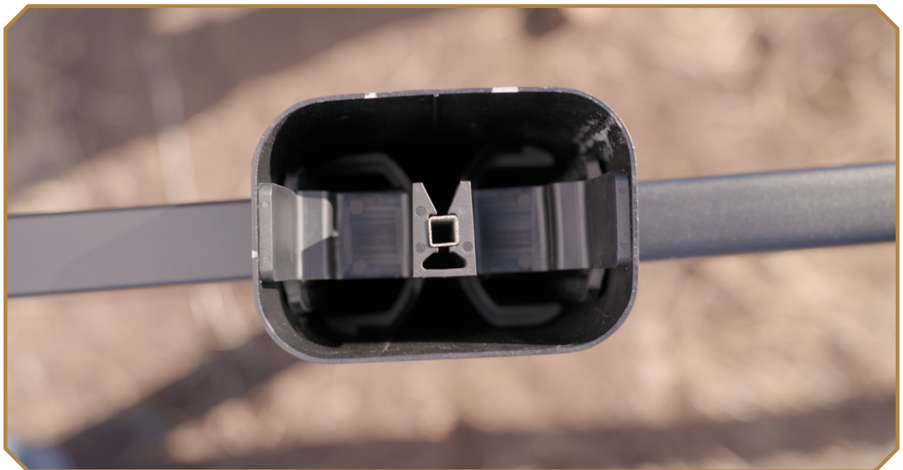
Above: Lock spacer being dropped in to line post. Below: Lock spacer resting on the inserted rails.
